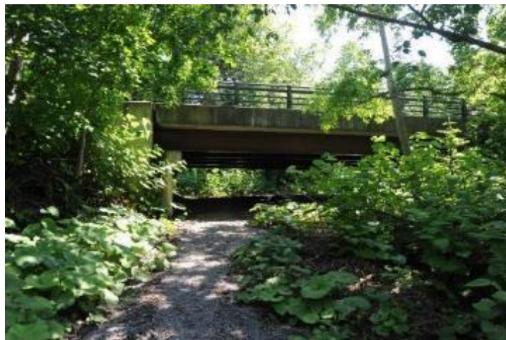
Figure 5 Monbetsu Bridge (Route 276)
