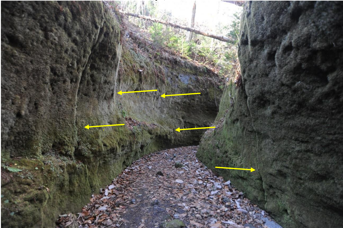
Figure 15 Joints found in the "Koke-no-kairo Gulley (Moss Corridor)"
