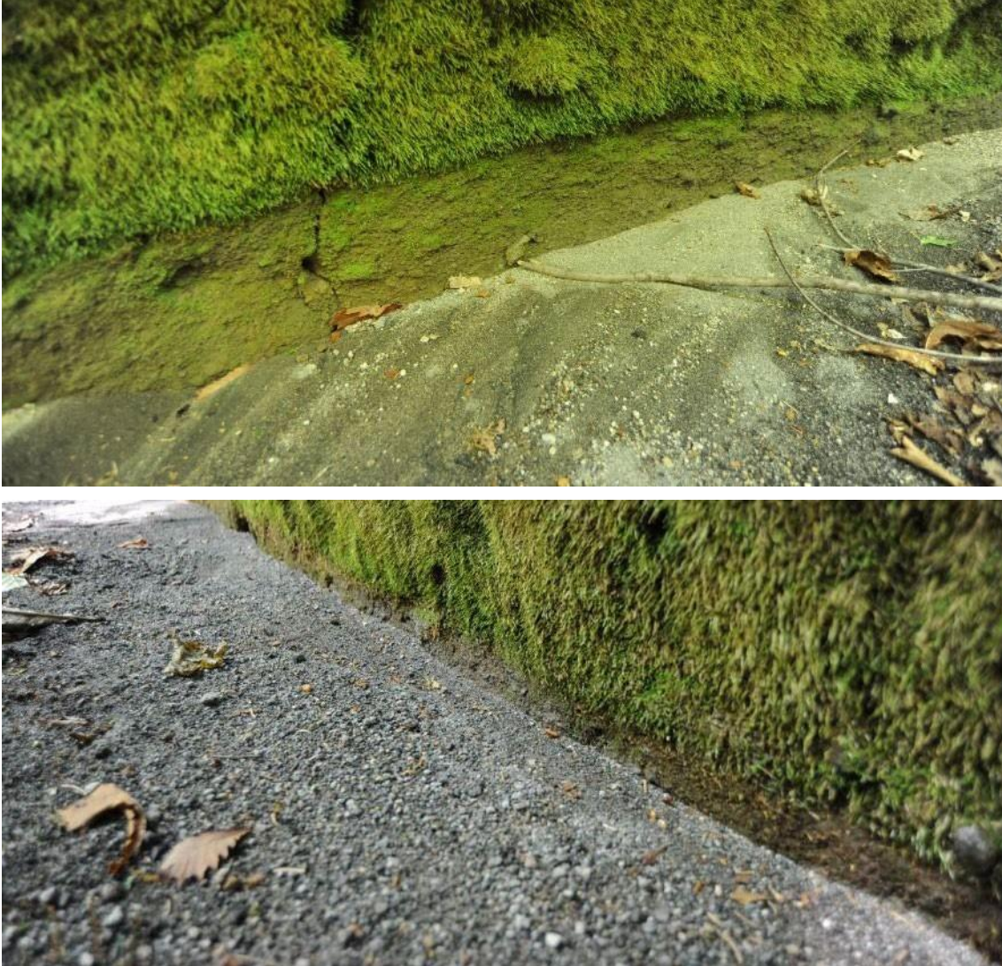
Figure 19 Deposition and Movement of Sediment (3)
