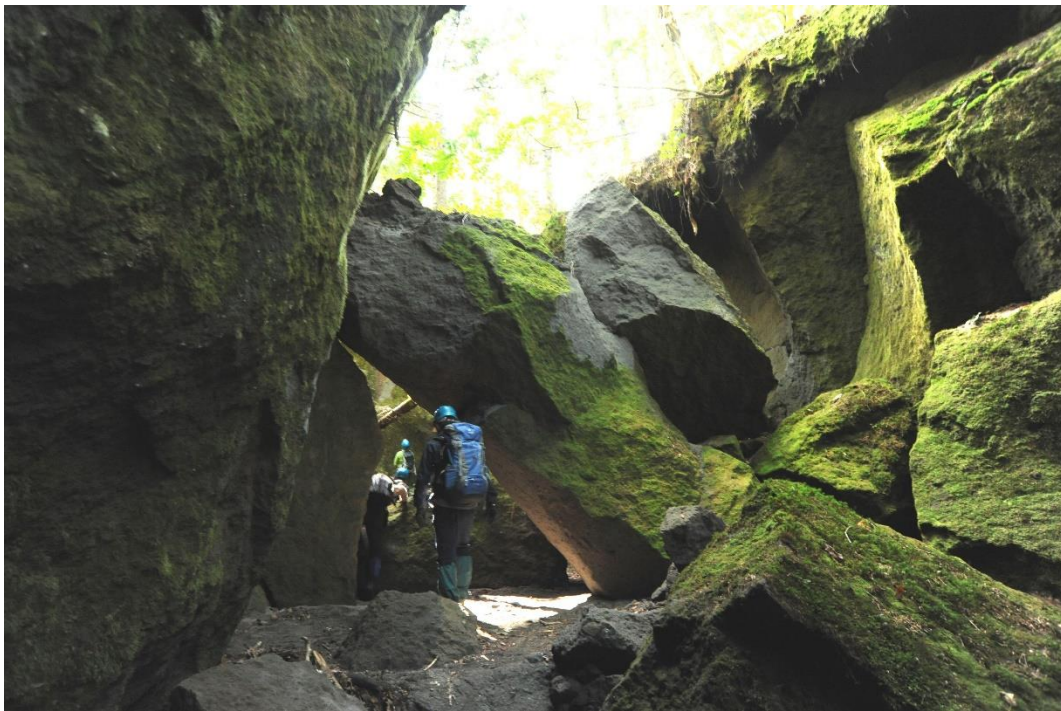
Figure 21 Large-scale rock slope failure
